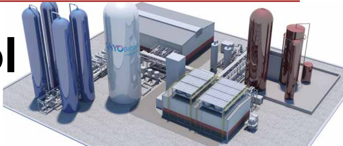
As a thermo-mechanical battery, energy is stored as liquefied air in tanks. When power is needed heat exchangers evaporate the liquid air, which expands through an expander-type turbine to drive a generator
